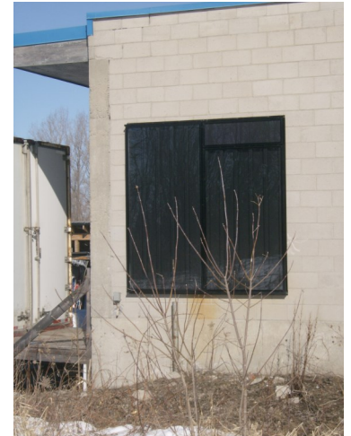
Thanks to Rideau Home Hardware for working with us to incorporate the solar thermal panels at the REAL Deal.
