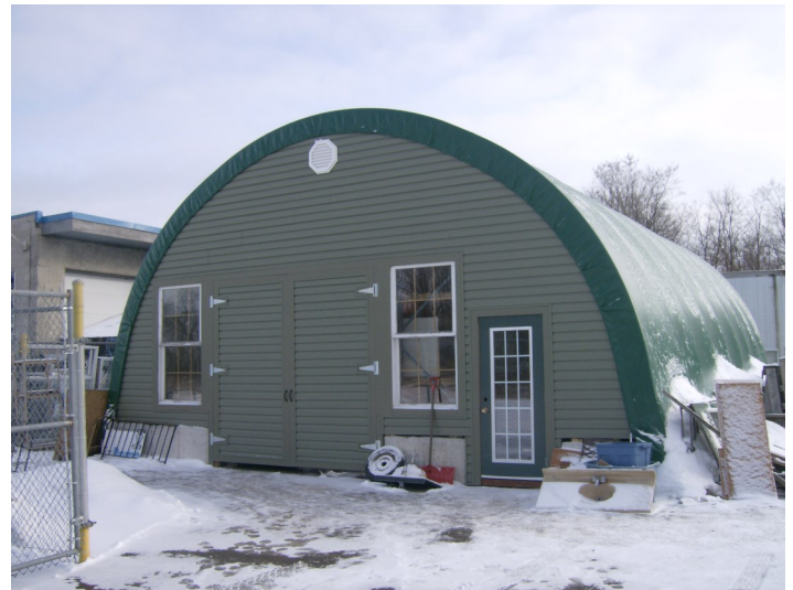
The two ends of the EZ Dome coverall behind the REAL Deal Store have now been enclosed. See REAL Deal News inside for more.
