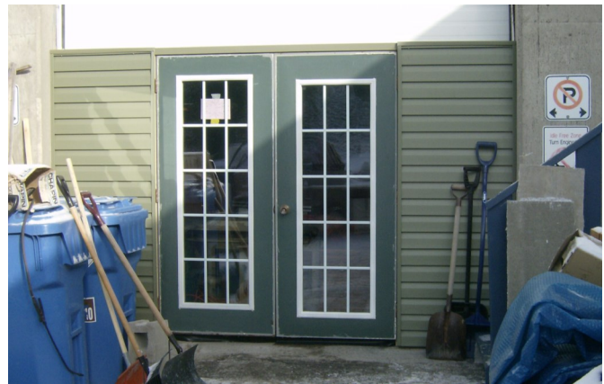
New doors into the store from the yard. Thanks to volunteer Bill Hamilton for this major improvement.
