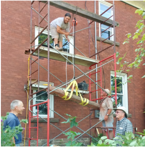
Stone window sills being lowered from tearout home at 140 Elmsley Street.
