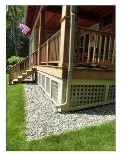
2. Fill the trench with  $\frac{1}{2}$ " -1 $\frac{1}{2}$ " crushed stone. The front and sides of the trench may be edged with stone or with pressure-treated lumber to hold the stones in
